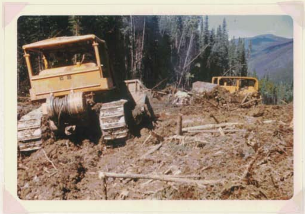
Photo 5. Road construction in vicinity of D.H.-9. Two "Cats" always worked together in muddy areas.
