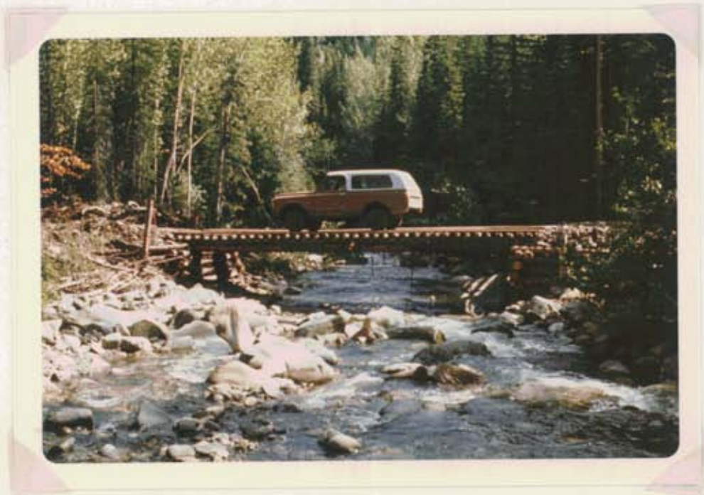
Photo 8. Seven Mile Creek bridge, all timber construction, decked with 3"x12" planking.
