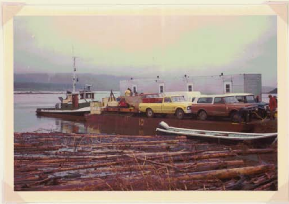
Photo 1. Equipment being loaded on barge at MacKenzie for towing to Carbon Creek. June 15, 1971
