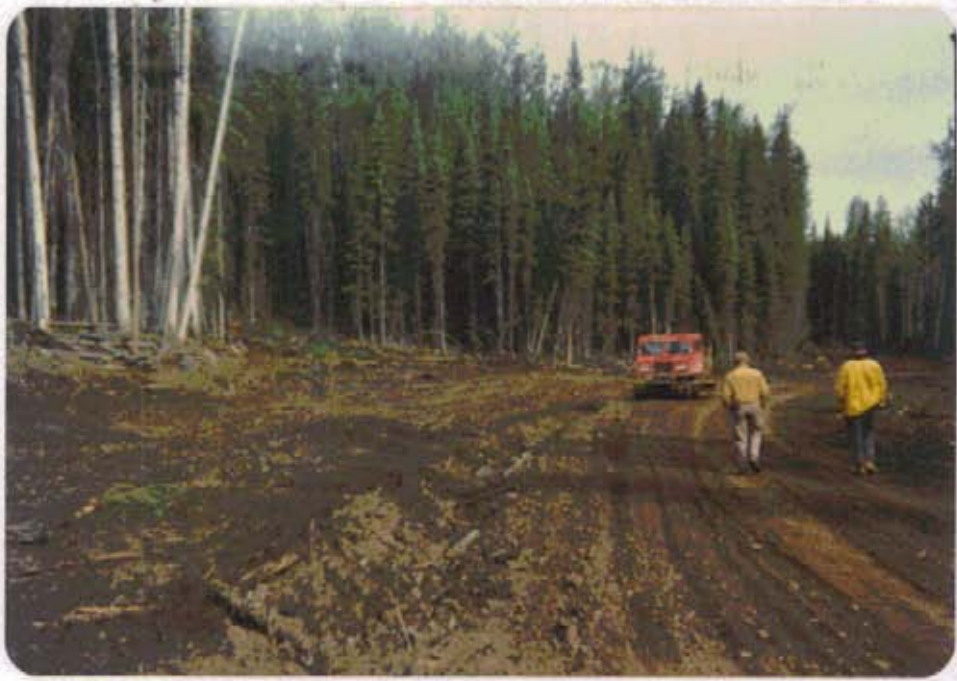
PHOTO 5: A cleared area along the main road just south of camp before seeding.
