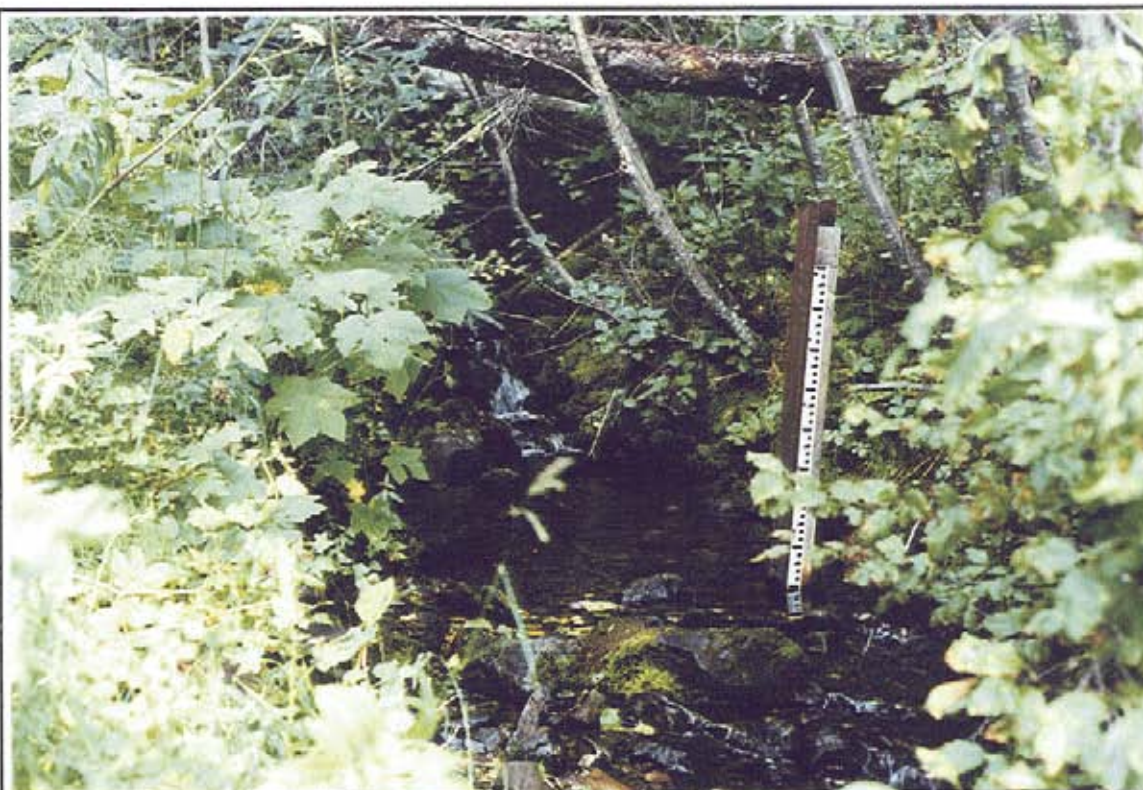
Trib 1 50m upstream of confluence and 120m downstream of road culvert. August 30, 1996.
