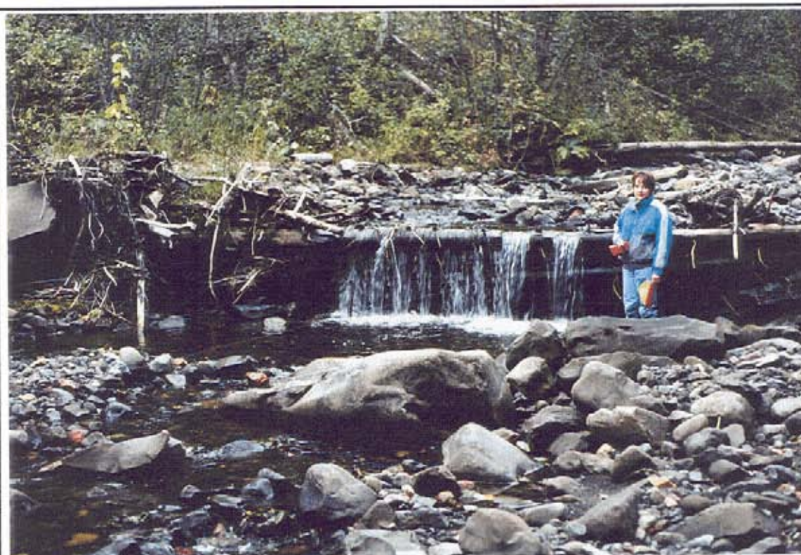
Willow Creek 172m above Trib 2 showing 1.4m obstruction. September 26, 1996.
