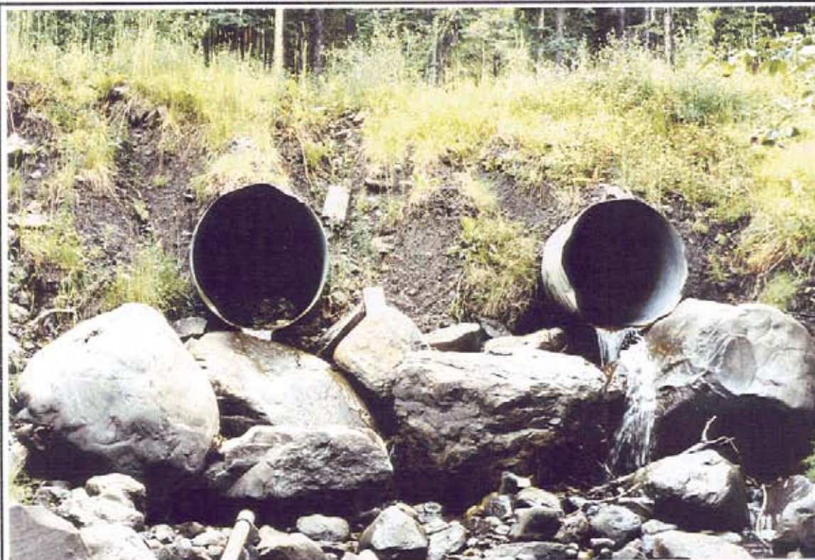
Trib 2, culverts at forest service road. August 30, 1996.
