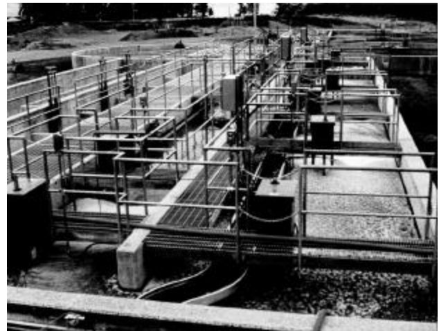
Photo courtesy of Turborator/Aquaplant Construction
