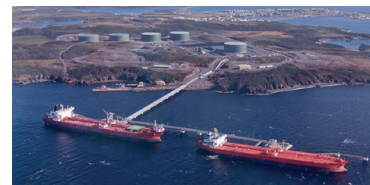
Newfoundland Transhipment Terminal serving the Hibernia Field
