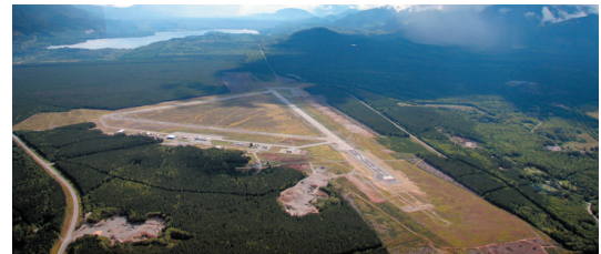
Terrace Airport Lands
