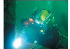
Coded wetwelder/ diver repairing marine structure
